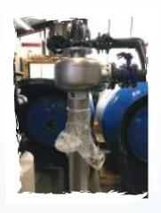
**Separator filter**Coarse filtration at 100 micron.
