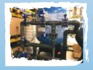
AFG system has been designed for a continuous flow and sufficient, a backwash is provided every 24-48h. The free volume required for this phase is 40%. The interval will be confirmed during commissioning. The different steps of this filter cleaning will be done automatically.
